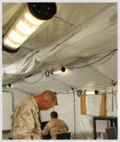
Pelican's new 9500 Shelter Lighting System (SLS) uses 24 tough LED lamp modules to instantly switch from white to night vision-safe red light. Personnel can perform command and control duties while maintaining natural night vision and also reduce exposure to the enemy.
